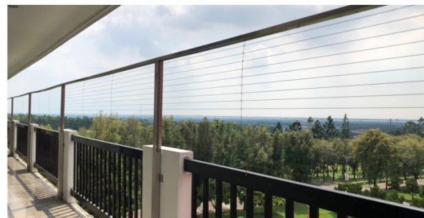
▲ Install fall prevention facilities on higher floors.
