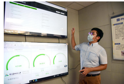
▲ Energy monitoring system of the Green Energy Light House
