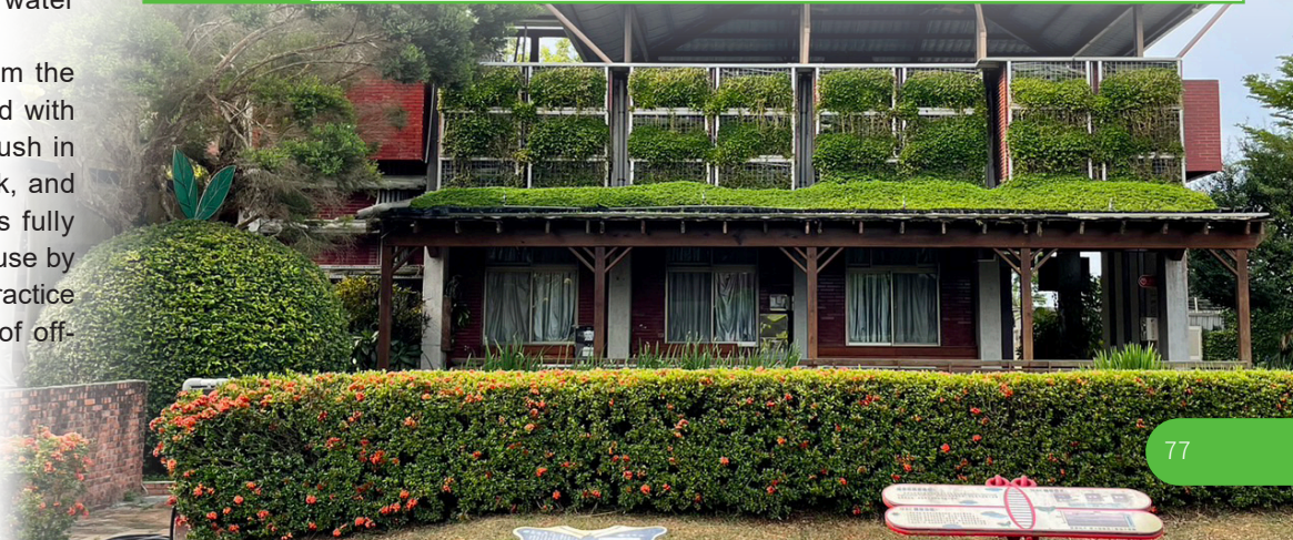
► Rainwater Harvesting System
