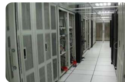
Hot aisle and cold aisle airflow system
